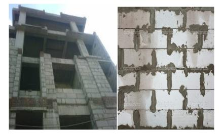
ACEBLOCK Premium is a high quality block fixing mortar designed to provide superior chemical anchoring between porous bricks. It is a specially formulated cementitious ready-mix adhesive to be mixed with water at site and used as thin bed adhesive for bonding light weight, aerated and all kind of building blocks. It can also be used to fix the tiles on wall made with similar blocks.
