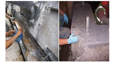
ACECOTE Epoxy bonding agent is a 100% solid, moisture-tolerant epoxy system designed to increase the bond between freshly-placed repair mortars or concrete mixes and existing concrete. It consists of pre-weighed Part A and Part B in pail. It is a high abrasion and impact resistant coat and has very good adhesion to concrete surface, plaster and all kind of metal.
