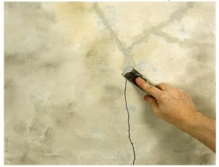
High performance acrylic based crack filler paste used for sealing or repairing internal and external cracks in plasters or masonry surfaces. It is a highly flexible yet tough, non-shrink crack filler used to fill cracks up to 5mm. It has very good adhesion property over all type of plastered wall or masonry works.
