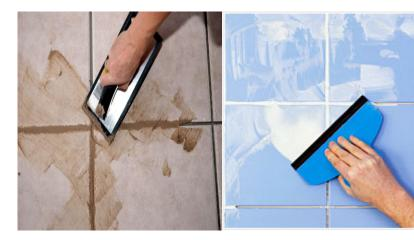
ACEMIX Grout admix is a high quality, milky white, latex based additive designed for use with ACEGROUT/AQUAPROOF Cementitious grout. ACEMIX Grout Admix is used in place of water to provide flexibility to the system after curing.
