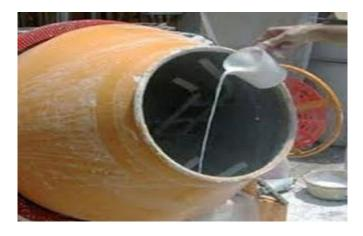
Aceproof IWP is high performance super plasticizing and water reducing admixture prepared with blending of selected superior grade ingredients under supervision from experts. It is recommended to add 200ml-500ml dosage per 50kg cement.
