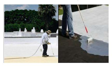
ACEPROOF Ener-G'guard - High performance acrylic elastomeric coating has excellent elongation and can maintain a watertight seal while the roof expands and contracts for certain extent. It has high resistance to organic growth and has UV resistance properties too. ACEPROOF Ener-G'guard - High performance acrylic elastomeric waterproofing coating saves money on cooling costs by reducing the heat transferred to the inside of your building.
