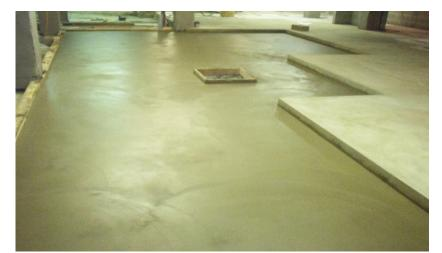
ACECREED - Concentrated is a cementitious screeding material prepared by using high performance chemical ingredients, premium cement and supplementary binders. It is heavy load bearing, self-curing screed designed for use with required proportion of water and aggregates at site. It is also designed for mix with a small proportion of ACEMIX TBL for flexibility and improved performance.
