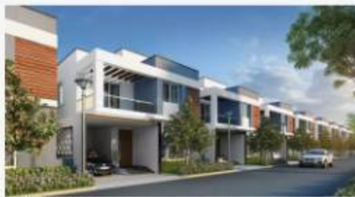
Project: Nambiar Ellegenza, Bangalore Product Used: 120 MT Acefix 3 Star, 20 MT Acefix 7 Star, 20 MT Acepoxy Epoxy Grout
