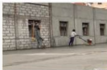
Project: Amirtha Viswa Vidhya Peedam, Chennai Product Used: Acefix Tile Adhesives, Acepoxy Epoxy Grout, Acefinish Wallcare Putty, Acefinish Wall Primer
