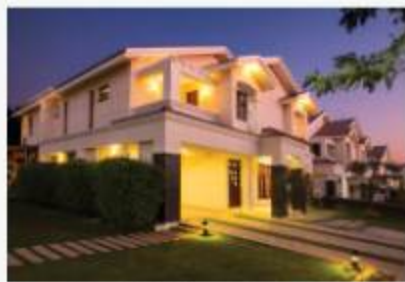
Project: Nambiar Bellezea, Bangalore Product Used: More than 200 MT Acefix 3 Star, 50 MT Acefix 7 Star, 20 MT Acefix 9 Star White, 10 MT Acepoxy Epoxy Grout
