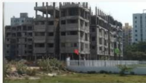
Project: Marutham Group Flats, Chennai Product Used: Acefix Tile Adhesives
