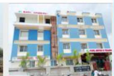
Project: Patil Hospital, Ilkal Product Used: Acefix 3 Star, Acefix 5 Star, Aceoxy Epoxy Grout
