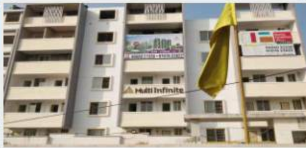
Project: Multi Infinite, Bangalore Product Used: Acefinish Wall Primer, Acefix 3 Star, Acepoxy Epoxy Grout
